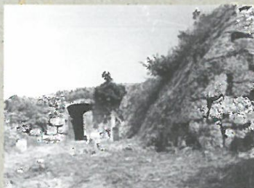
Before repair [ Photo taken in 1973 ]
