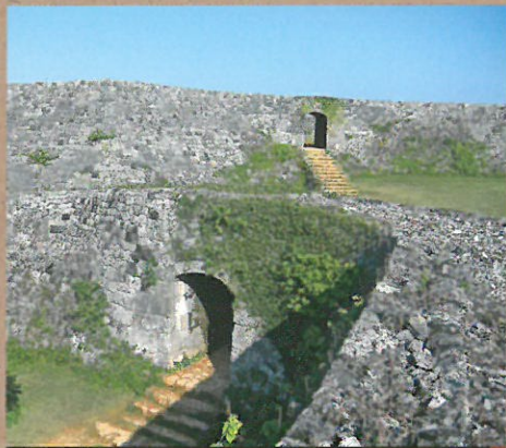
① Two arched stone gates
