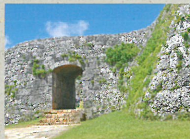
After repair [ Photo taken in 2014 ]
